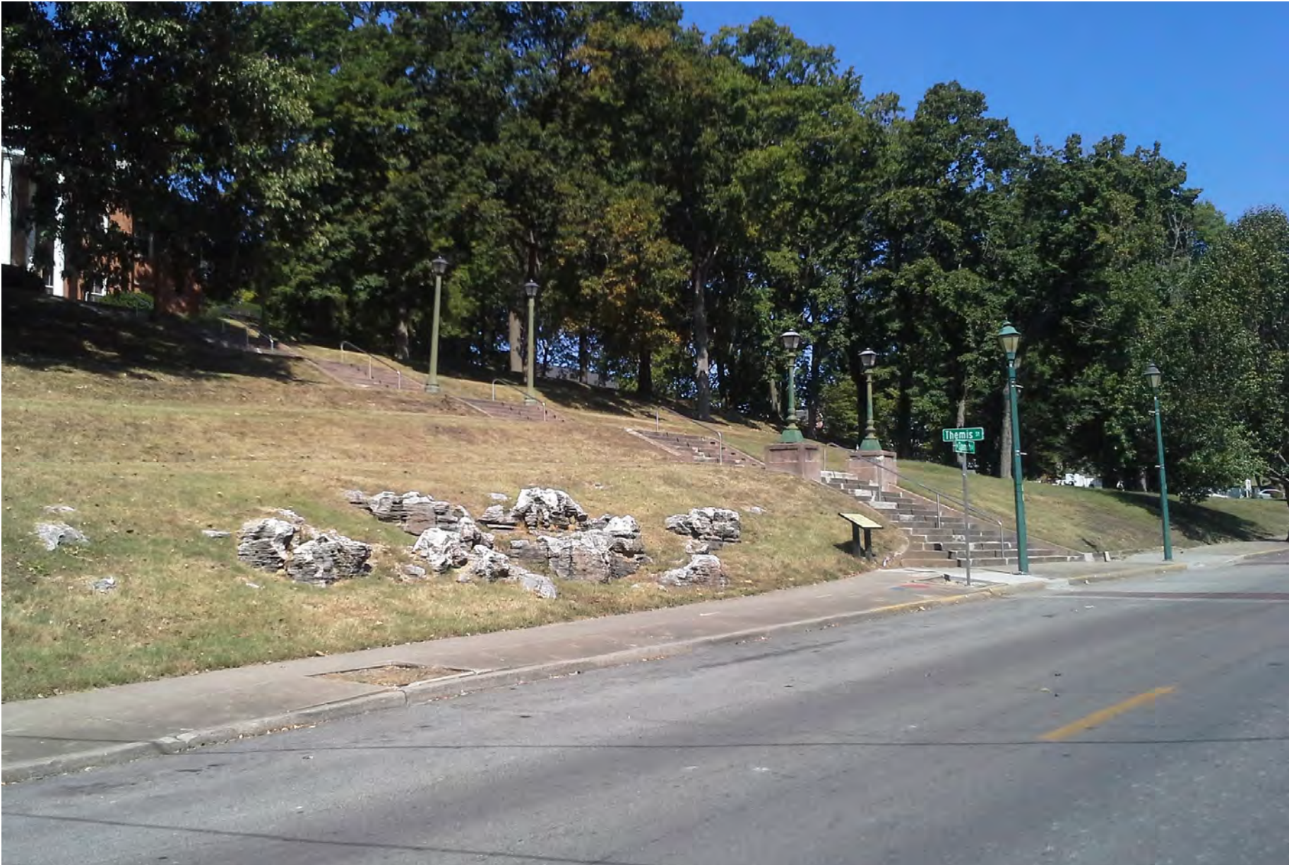
View of the existing conditions along North Spanish Street, on the east side of the courthouse lawn. (View to the northwest.)
